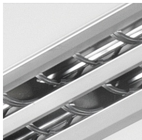
Detail of supply air slot
