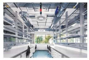
Air management systems in laboratories must be able to adapt quickly and precisely to prevailing air conditions. Equipment used such as safety workbenches and fume cupboards lead to constantly changing conditions in the room due to their variable exhaust air volume volume.
