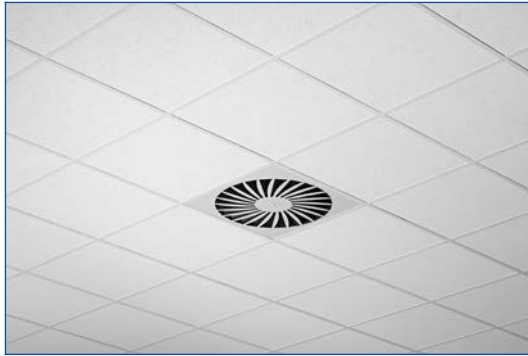
Installation in T-bar ceilings
