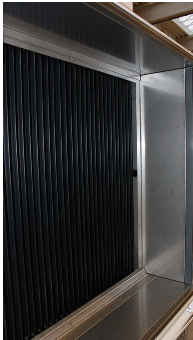
Inner skins made of stainless steel
