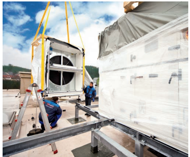
Delivery and installation of a weatherproof X-CUBE
