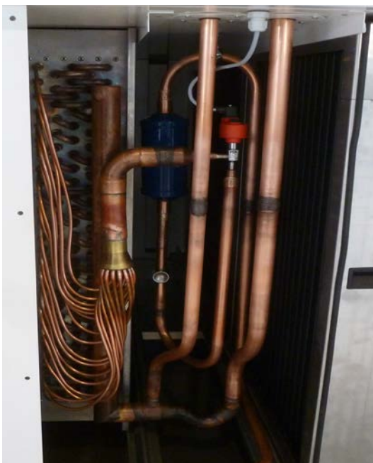
Venturi-type distributor in the evaporator
